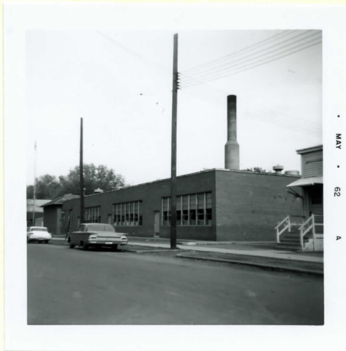
Rear View of North Side of North Wing
