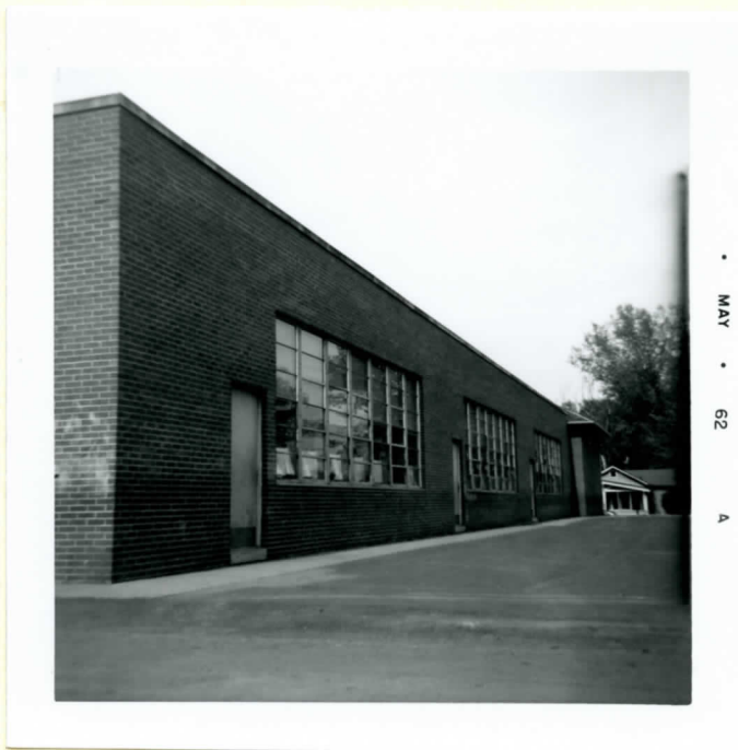
View of South Side of South Wing
