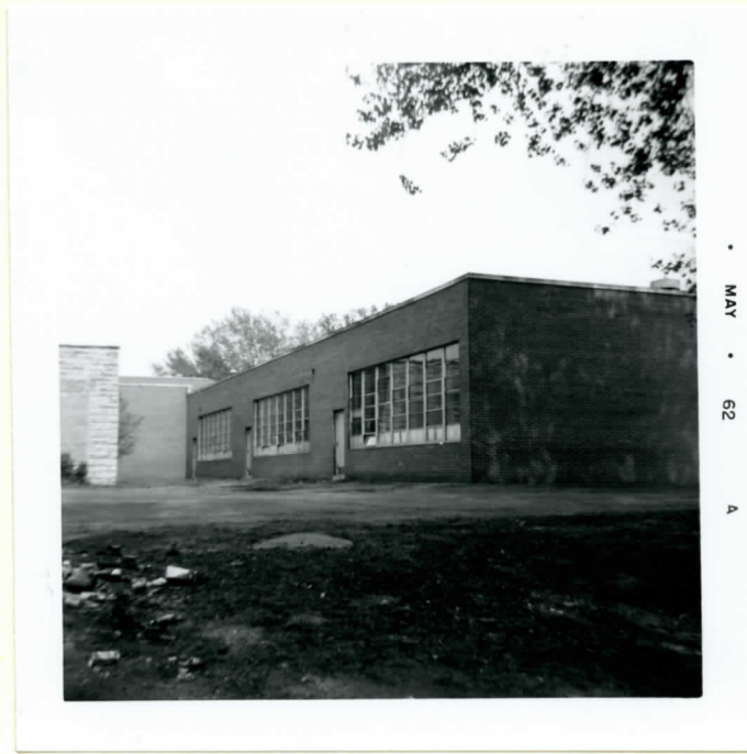
View of North Side of South Wing
