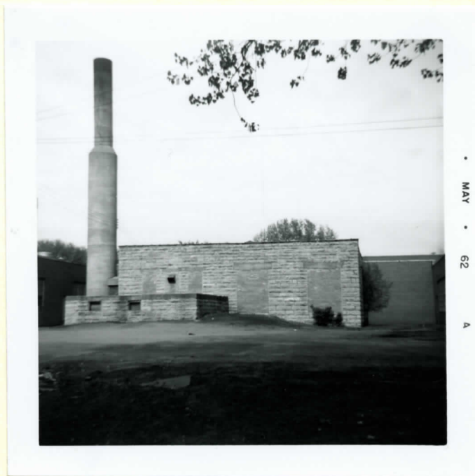
View of Boiler Room
