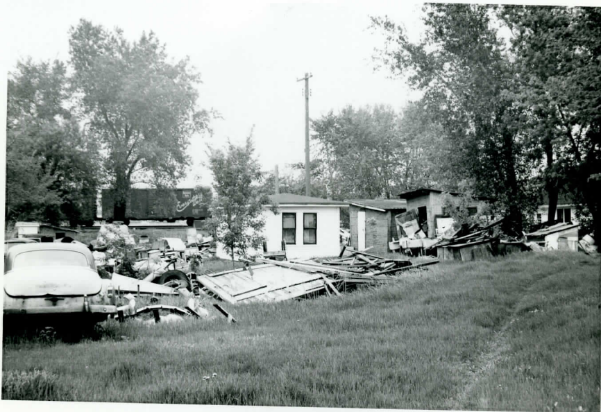
VIEW OF IMPROVEMENT & OUT-BUILDINGS ON NORTH PORTION OF LOT FOUR
