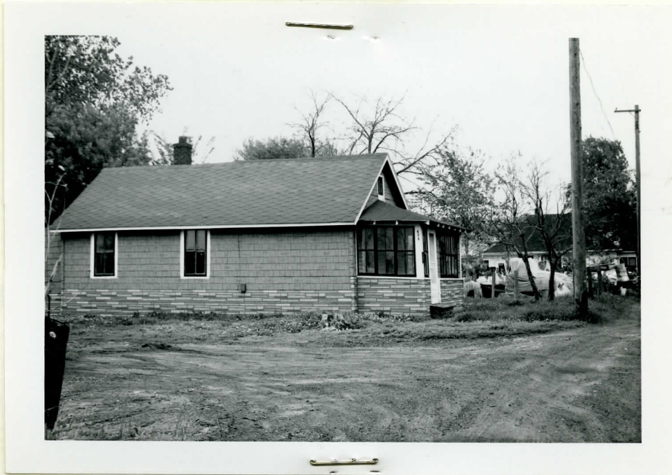
SIDE VIEW LOOKING TO THE EAST OF HOUSE LOCATED ON SOUTH PORTION OF LOT 10
