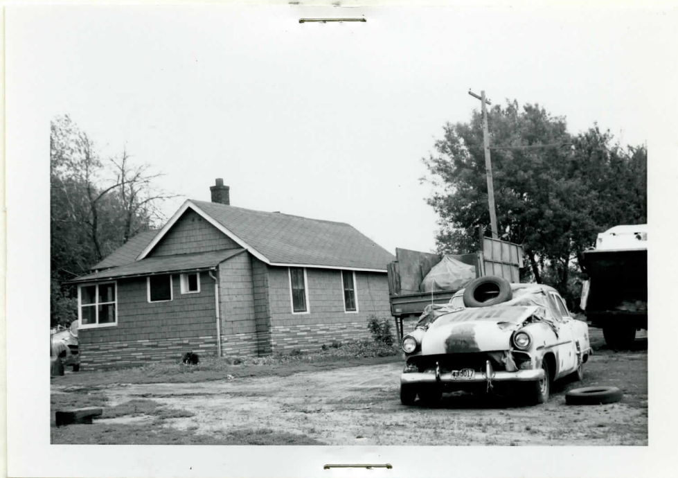
VIEW OF REAR OF HOUSE LOCATED ON SOUTH PORTION OF LOT 10
