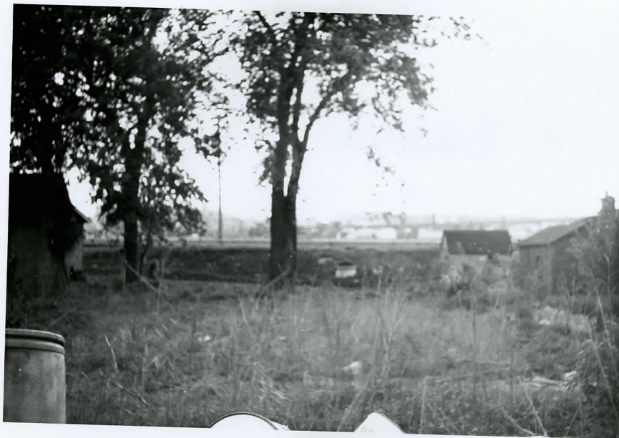
A VIEW OF LOT 9 LOOKING TO THE NORTH
