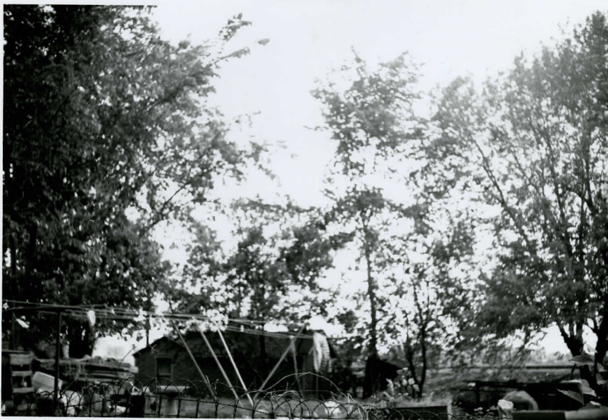
VIEW OF BUILDING AND LOT 8 LOOKING TO THE NORTH
