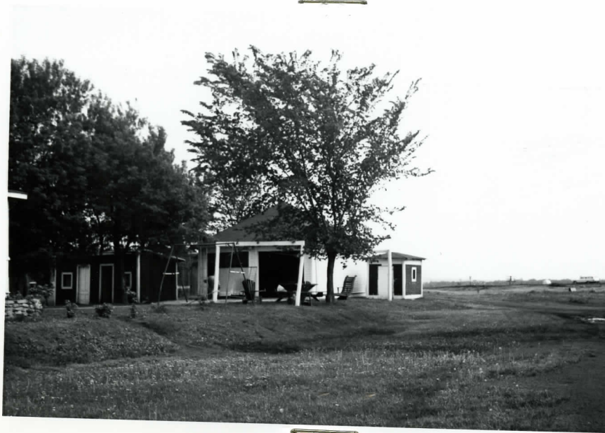
VIEW OF THE FRONT OF GARAGE AND SHEDS
