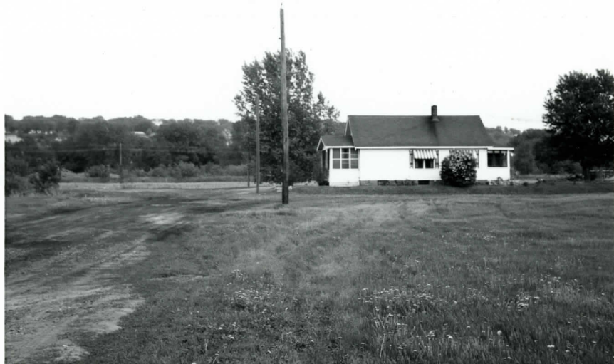
STREET VIEW LOOKING NORTH FROM NAGASAKI ROAD
