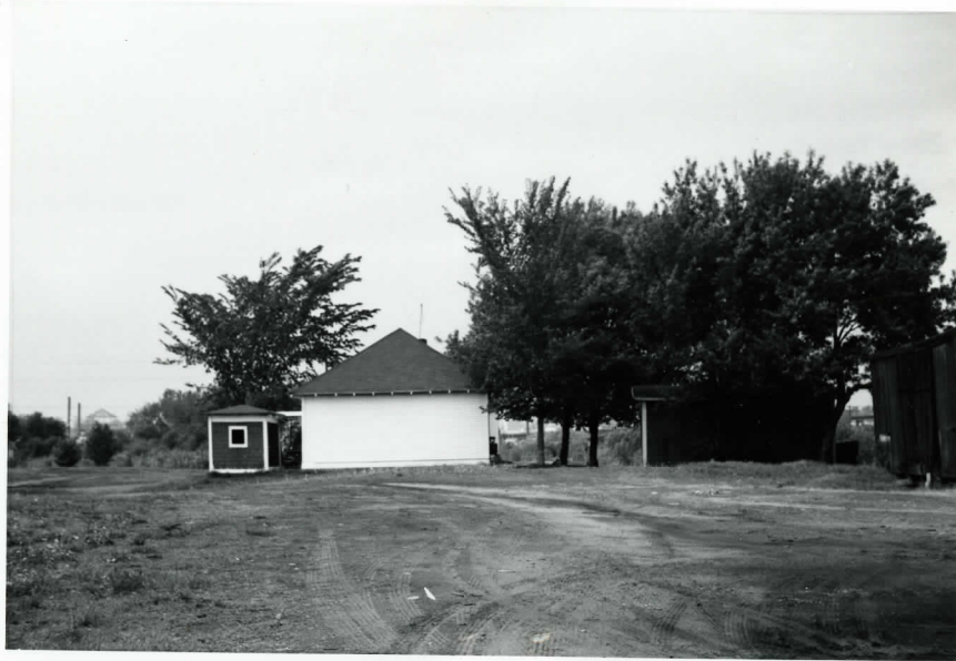
VIEW OF THE REAR GARAGE AND SHEDS
