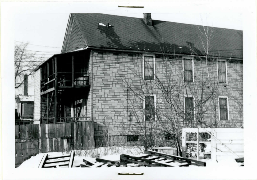
SIDE AND REAR VIEW
