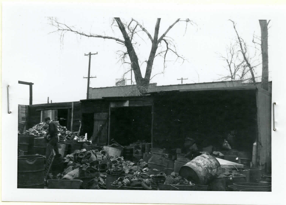
VIEW OF REAR
