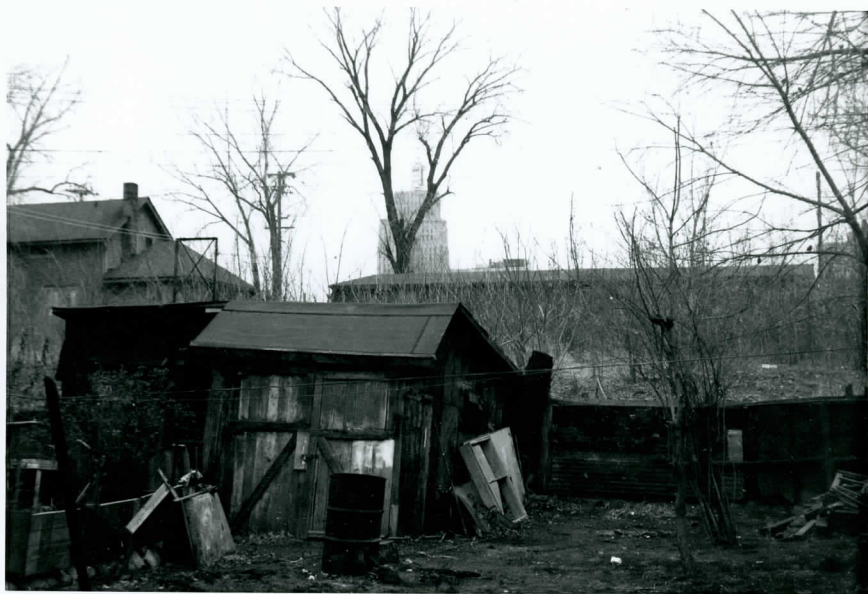
View of Shed
