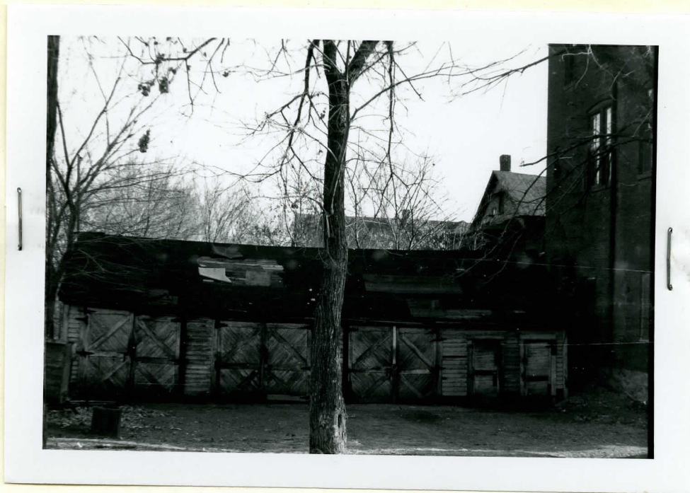
View of garages and sheds
