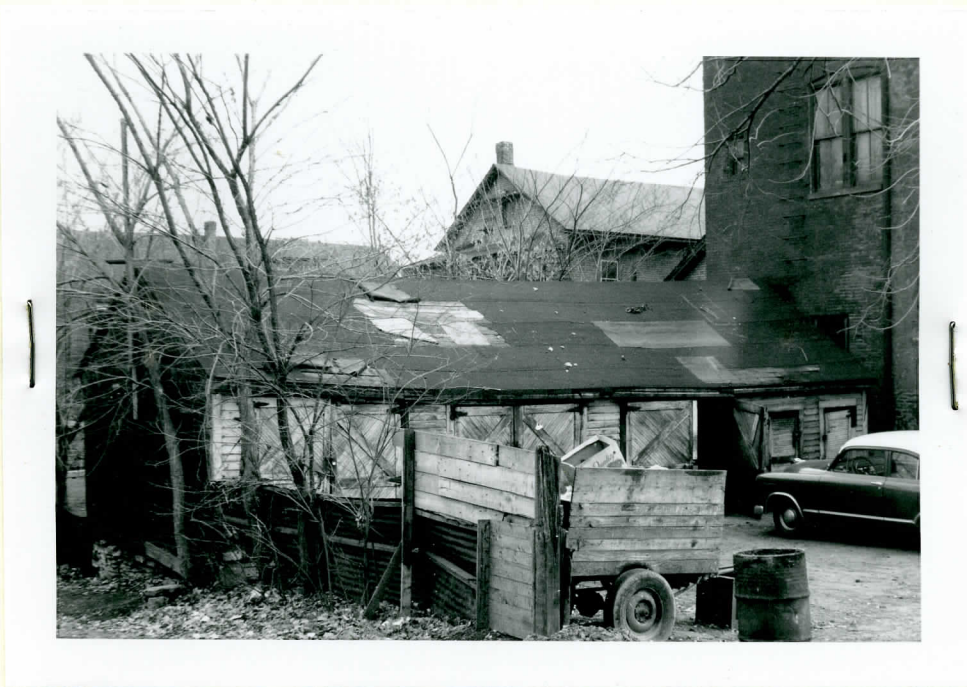
View of Garage + Rear of Main Building
