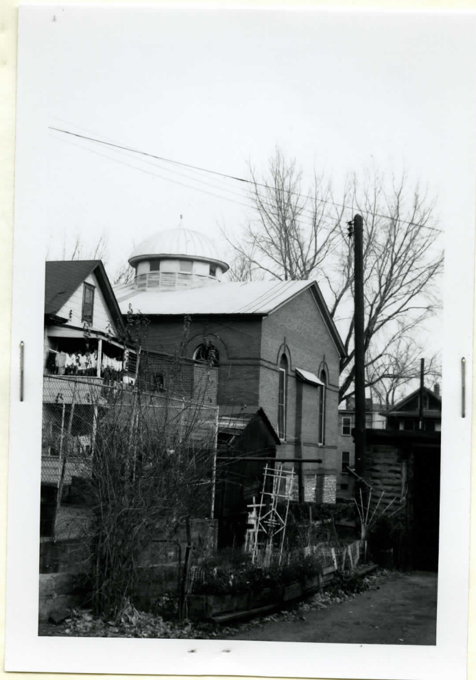
Rear View from East Side
