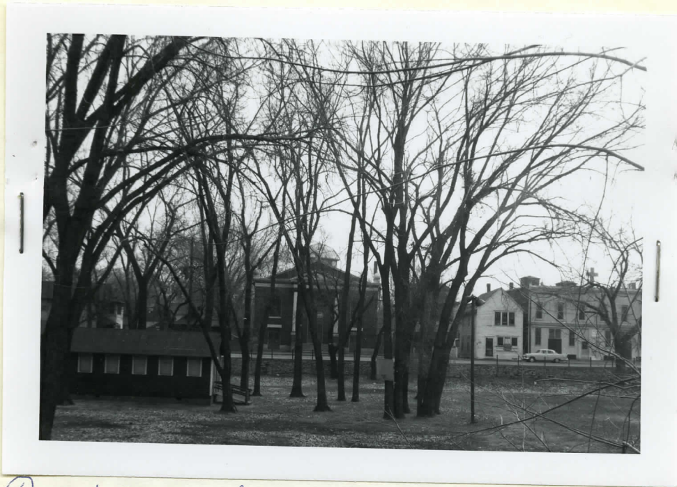
Front View from One Block North
