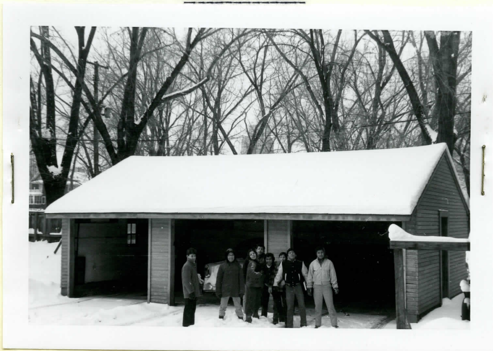
VIEW OF GARAGE
