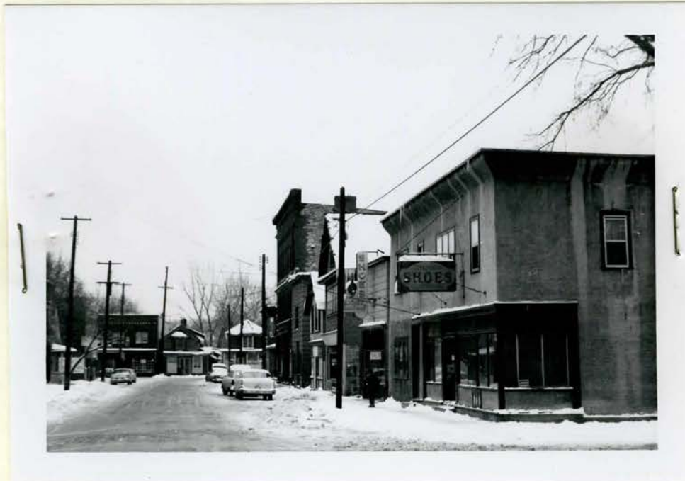
STREET SCENE SHOWING SIDE VIEW OF SUBJECT PROPERTY
