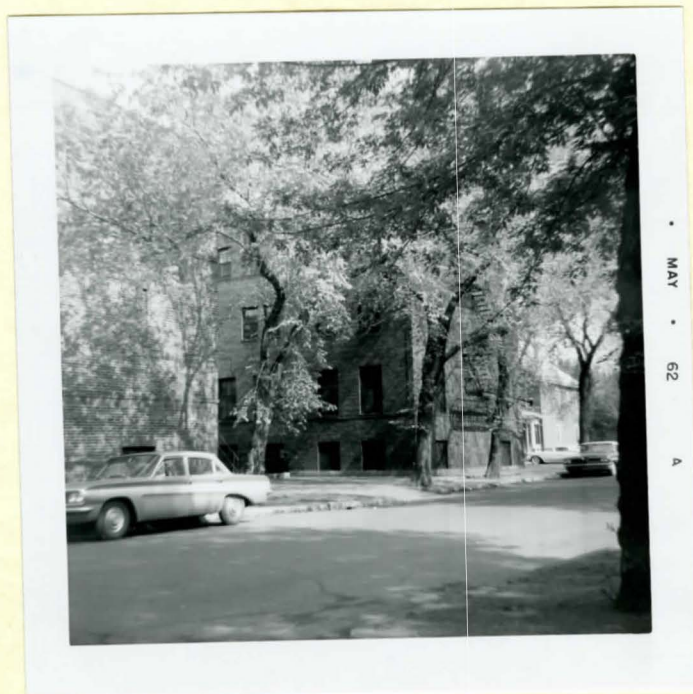
View of West Side of Building - Robertson Street
