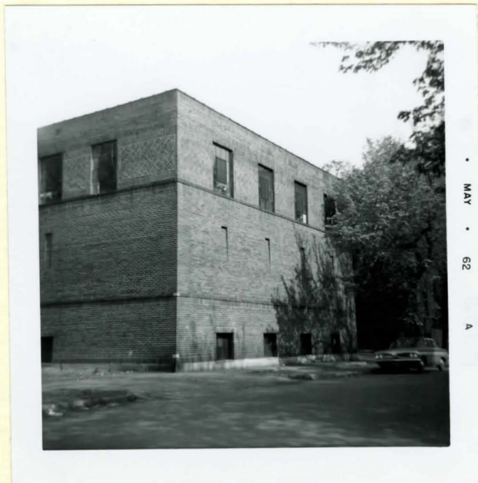
View of Rear Portion of Building
