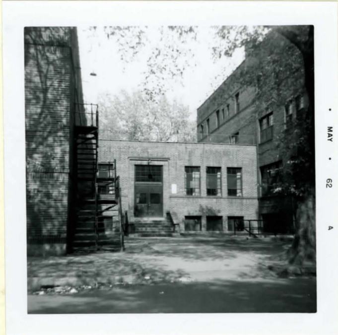
View of West Side of Annex
