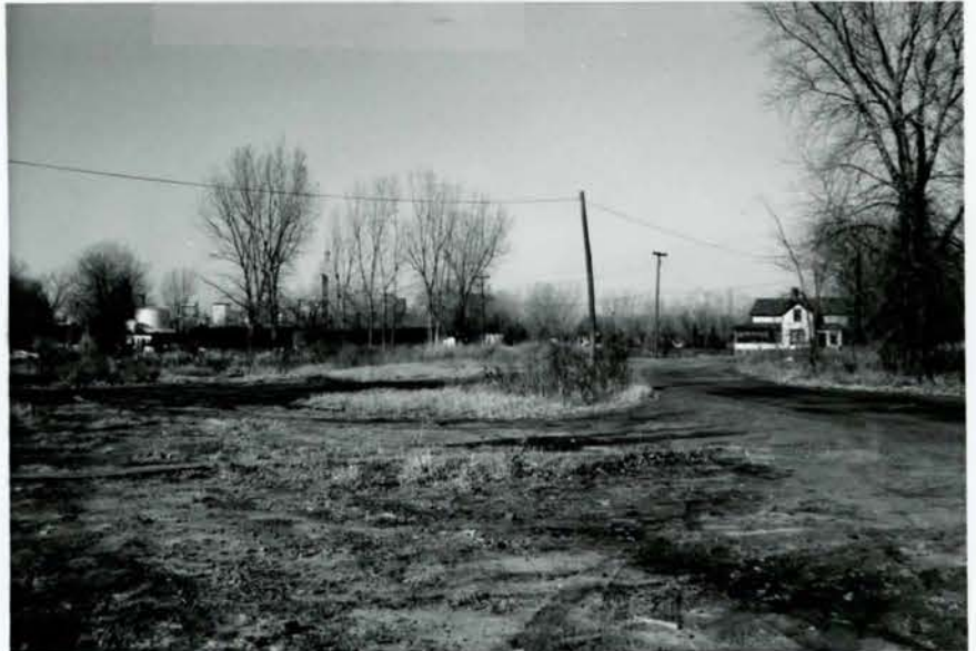
Looking N. W. ly at Block 10, Morrison's Addition
