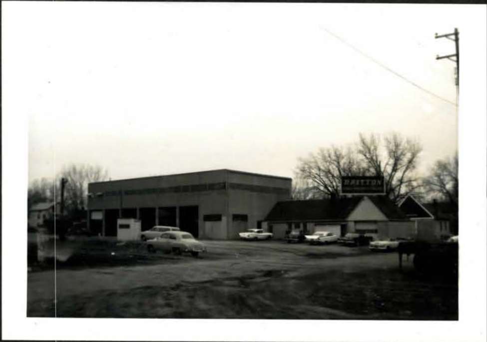
Metal Crane Shed - (Left) Office Building - (Right)
