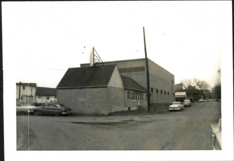
Office Building - (Foreground) Metal Crane Shed - (Rear)
