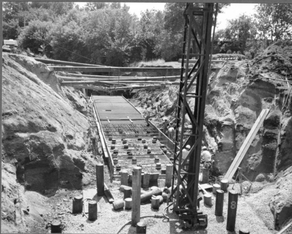
County Road 3 Box Culvert Foundation
