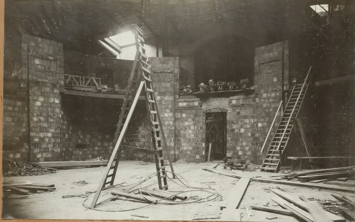
NO 211. MINNESOTA STATE CAPITOL. CASS GILBERT, ARCHT. VIEW IN HOUSE. NOV 18, 1902. HARRIS & WRIGHT PHOTO.
