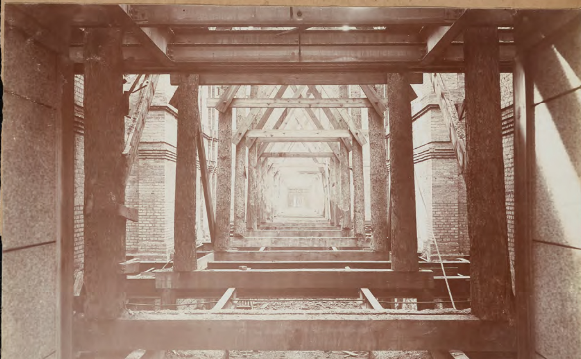
105. MAIN HALL LOOKING WEST. MINNESOTA STATE CAPITAL. CASS GILBERT ARCHT. MAY. 1, 1900. HANSBRO PHOTO.
