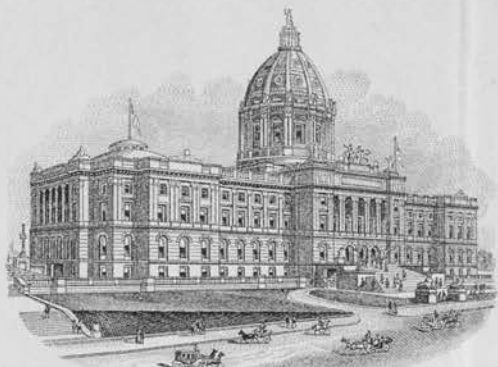
NEW STATE CAPITOL IN COURSE OF CONSTRUCTION.
