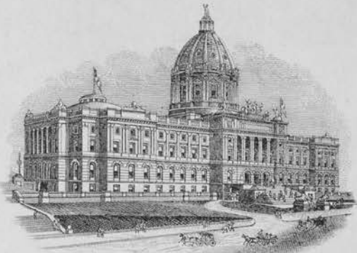
NEW STATE CAPITOL IN COURSE OF CONSTRUCTION. PHOTOGRAPH BY J. J. HANCOCK, ST. PAUL, MINN.
