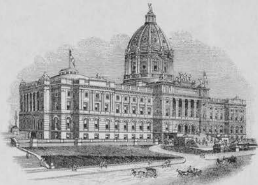
NEW STATE CAPITOL IN COURSE OF CONSTRUCTION. NEIGHBORHOOD LOCATED BY ST. PAUL, MINN.
