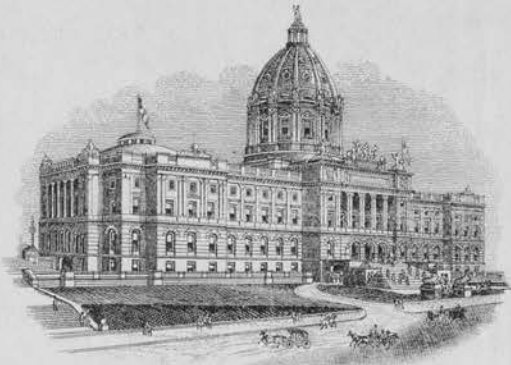
NEW STATE CAPITOL IN COURSE OF CONSTRUCTION
