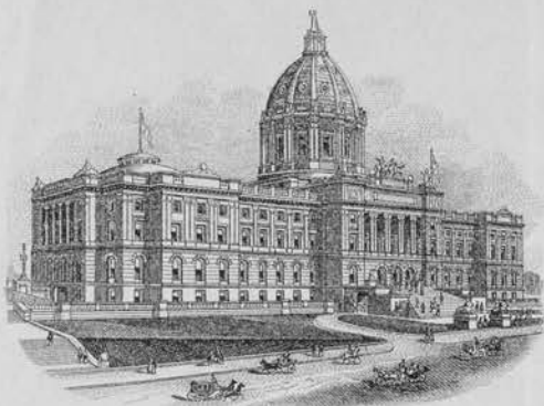
NEW STATE CAPITOL IN COURSE OF CONSTRUCTION.
