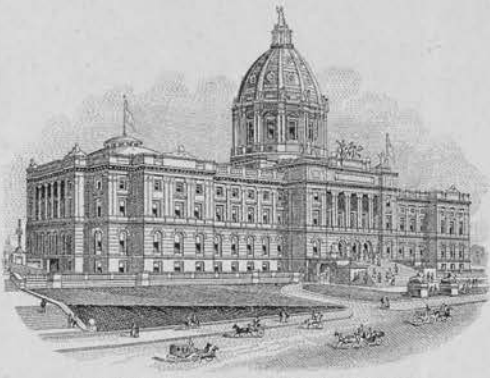
NEW STATE CAPITOL IN COURSE OF CONSTRUCTION.
