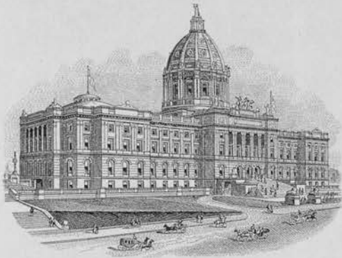
NEW STATE CAPITOL IN COURSE OF CONSTRUCTION.
