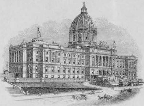
NEW STATE CAPITOL IN COURSE OF CONSTRUCTION PHOTOGRAPH BY J. H. ST. PAUL, 1899
