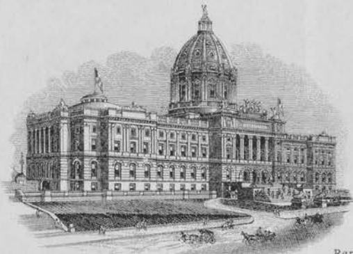
NEW STATE CAPITOL IN COURSE OF CONSTRUCTION. BY G. W. HARRIS, ST. PAUL, MINN.
