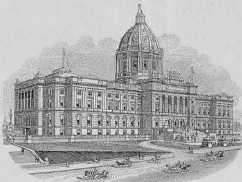
NEW STATE CAPITOL IN COURSE OF CONSTRUCTION.
