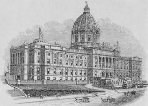
NEW STATE CAPITOL IN COURSE OF CONSTRUCTION PHOTOGRAPH BY LEO STADLER
