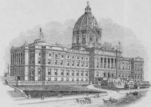
NEW STATE CAPITOL IN COURSE OF CONSTRUCTION. PHOTOGRAPH BY C. L. WILSON, ST. PAUL, MINN.
