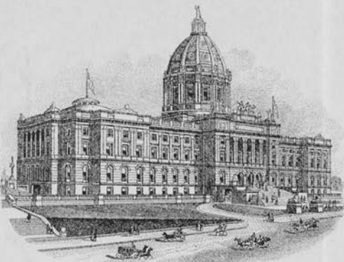
NEW STATE CAPITOL IN COURSE OF CONSTRUCTION.
