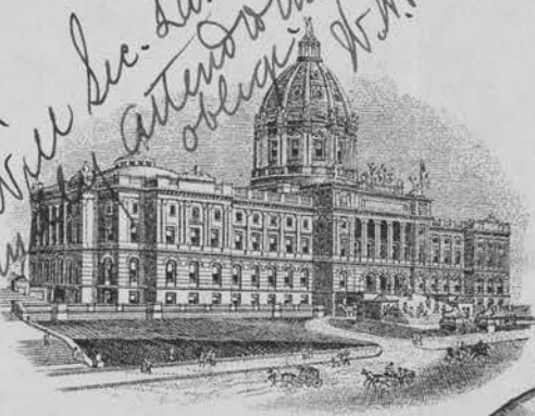
NEW STATE CAPITOL IN COURSE OF CONSTRUCTION
