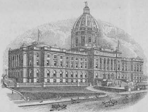
NEW STATE CAPITOL IN COURSE OF CONSTRUCTION.
