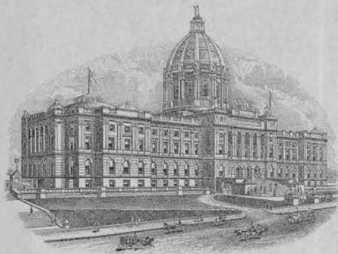
NEW STATE CAPITOL IN COURSE OF CONSTRUCTION.
