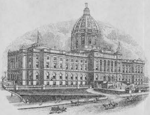
NEW STATE CAPITOL IN COURSE OF CONSTRUCTION.
