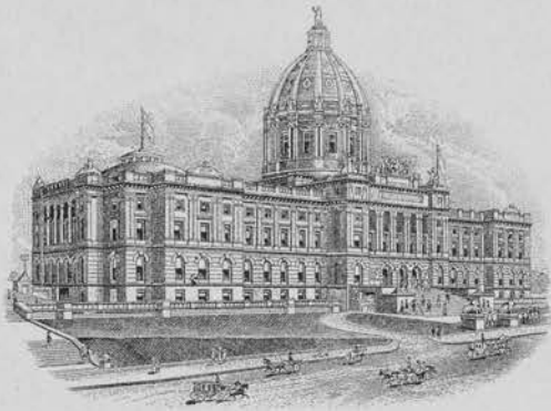
NEW STATE CAPITOL IN COURSE OF CONSTRUCTION.
