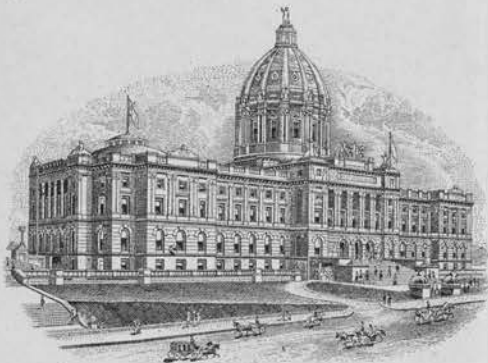
NEW STATE CAPITOL IN COURSE OF CONSTRUCTION.
