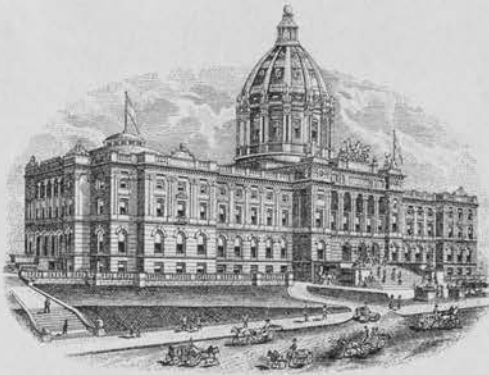
NEW STATE CAPITOL IN COURSE OF CONSTRUCTION
