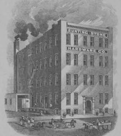
WHOLESALE AND SHIPPING WAREHOUSE 74,000 SQUARE FEET FLOOR SPACE 2012-2014-2016 BALTIMORE AVE.
