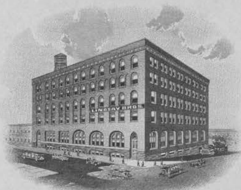
FOURTH AVENUE NORTH AND FIRST ST.
