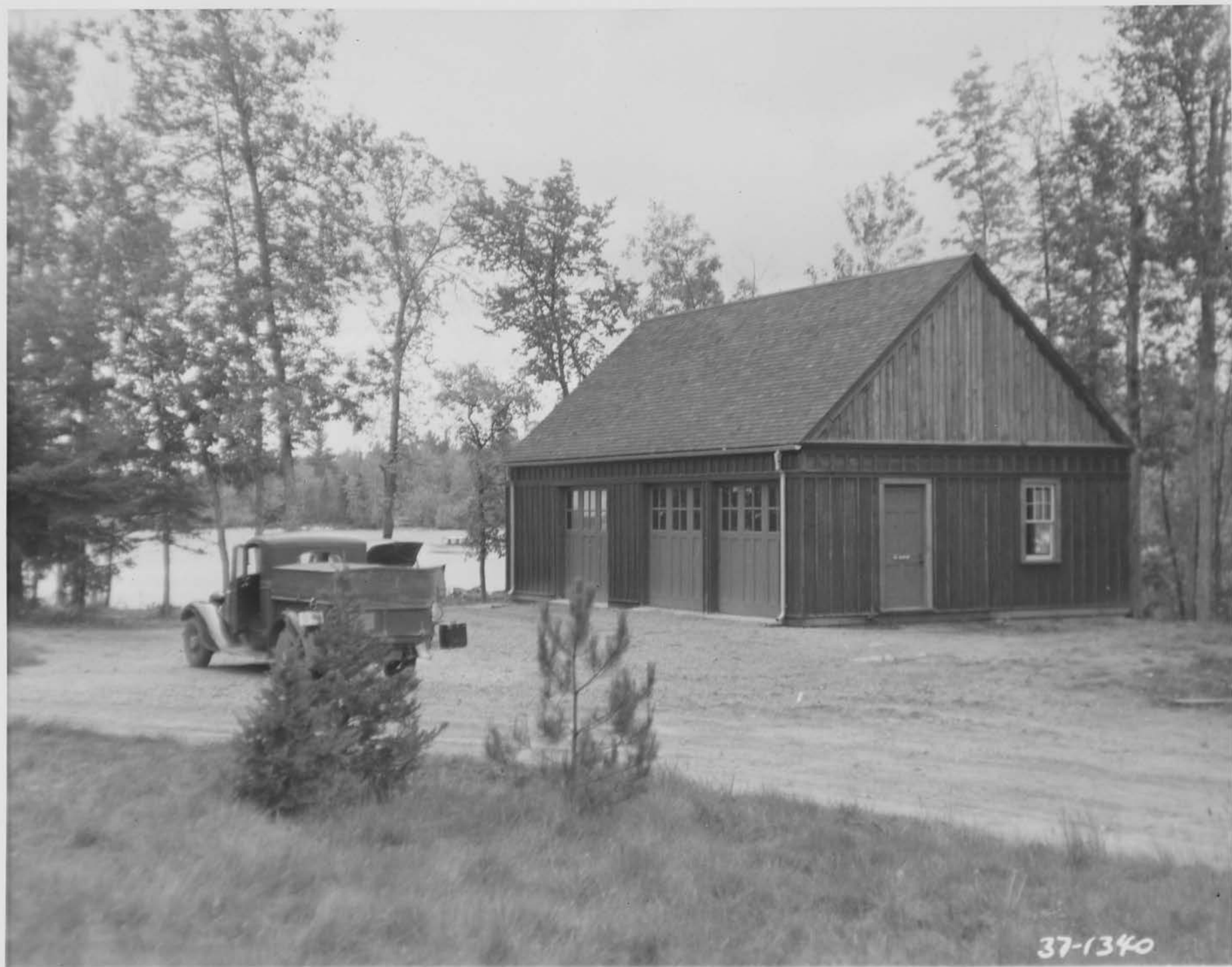
Garage on Kabetogama State Forestry Station Site, Dec. 21-69-71 Constructed by State C.C.C. Camp S-81, 1938.
