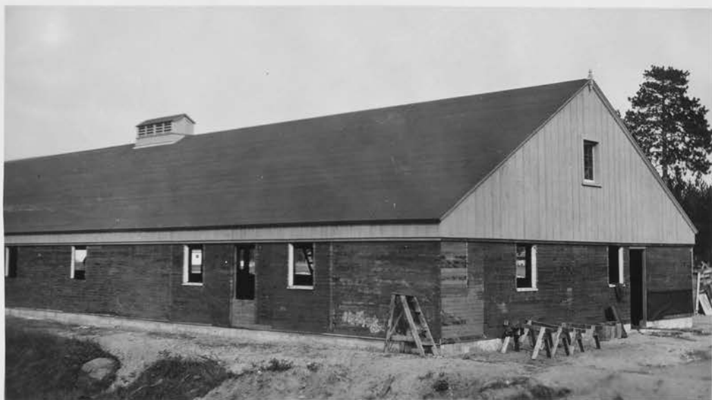
State C.C. Central office warehouse under construction by Camp S-54, Owen Lake. Grand Rapids, Minn Sept. 30, 1938.
