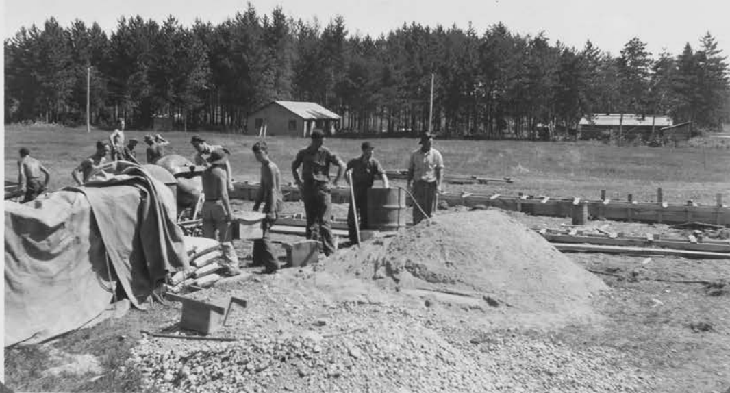
Mixing Concrete for Garage Foundation
