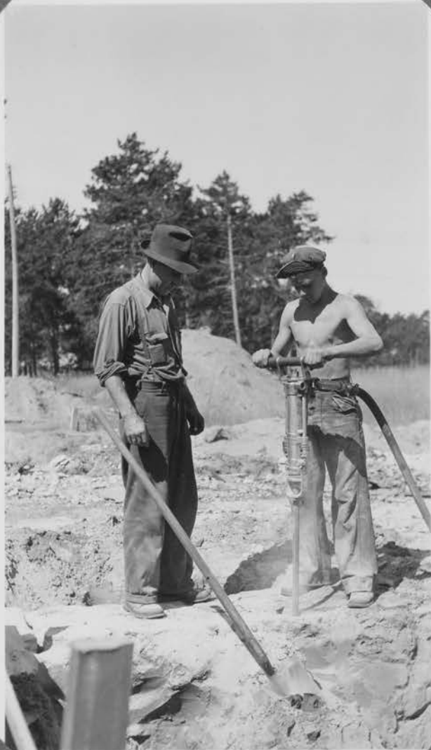
Air Hammer breaking up concrete for Warehouse foundation
