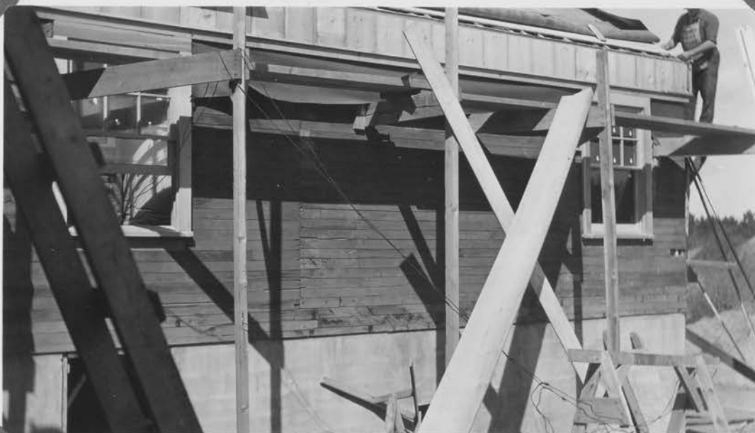
Showing Use of Salvaged Material for Frame
