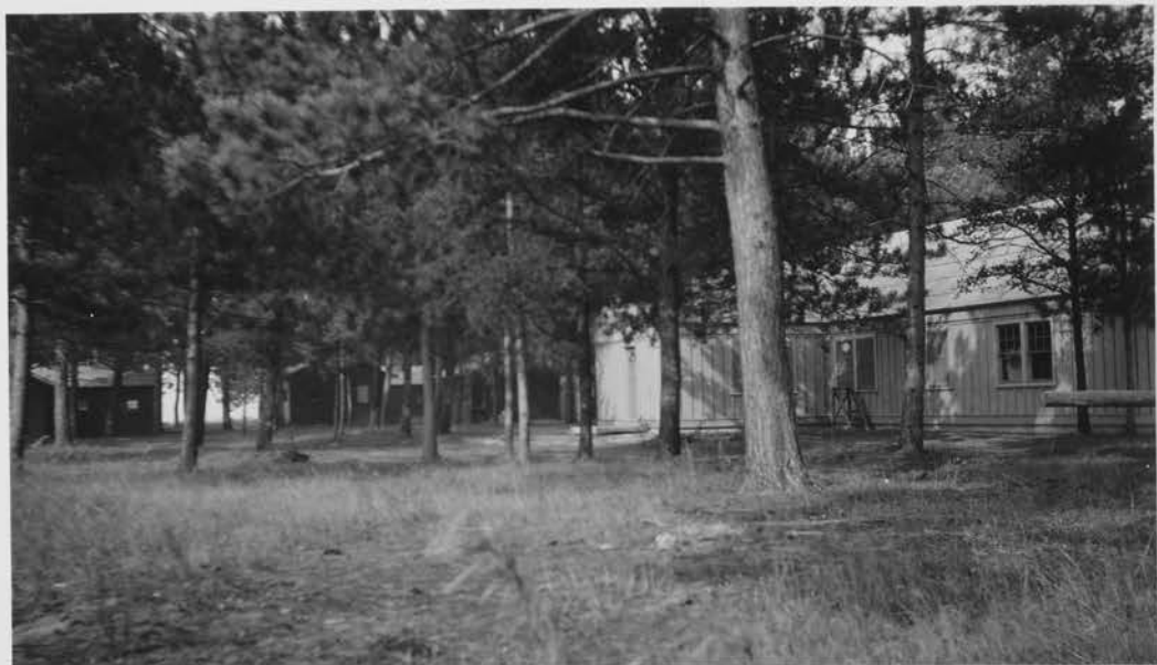
State ccc Office Building + Side Camp. Grand Rapids, Minn. Sept. 20, 1938.
