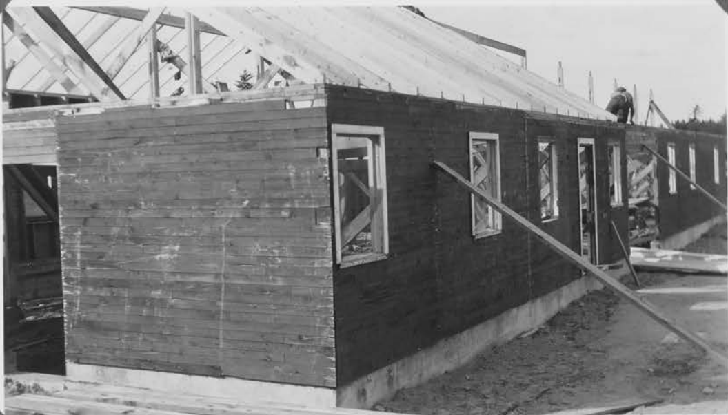
Warehouse Closeup of Salvaged Sections
