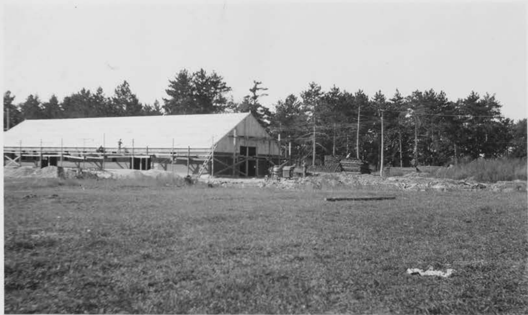
State ccc Central office warehouse under Construction by Camp S-54, Owen Lake. Grand Rapids, Minn. Sept. 20, 1938.
