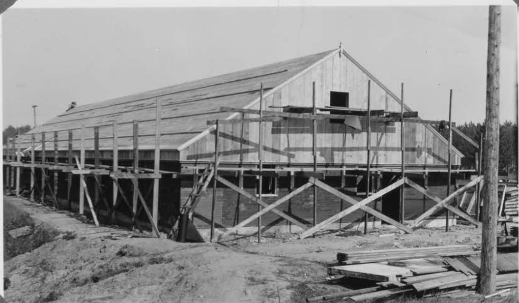
Warehouse South End
