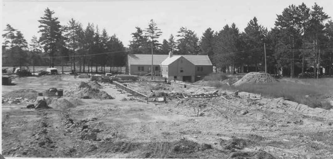
General View from Garage Warehouse Foundation in Foreground Administration Building in Background
