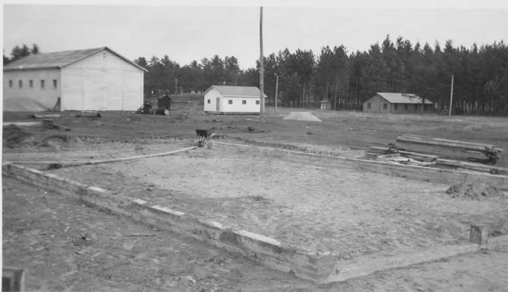
Completed Garage Foundation
