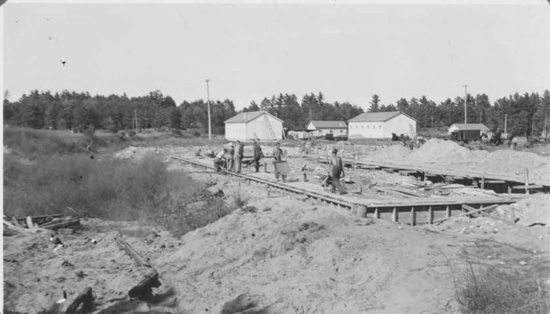
Pouring Warehouse Foundation View from Office
