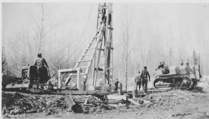
Pile Driver Rig. Camp S - Big Falls, Minn. Oct. 1938.
