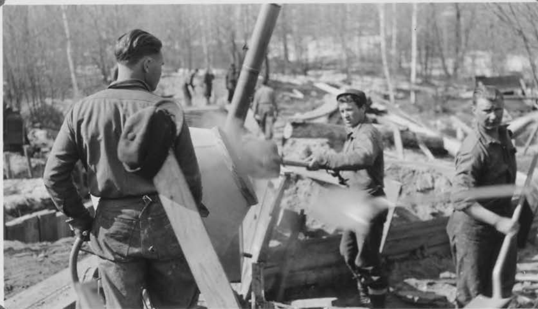
Loading Concrete Mixer
