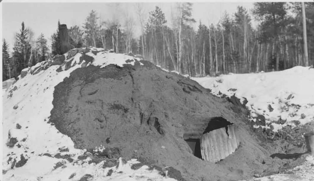
Heating Sand pile
