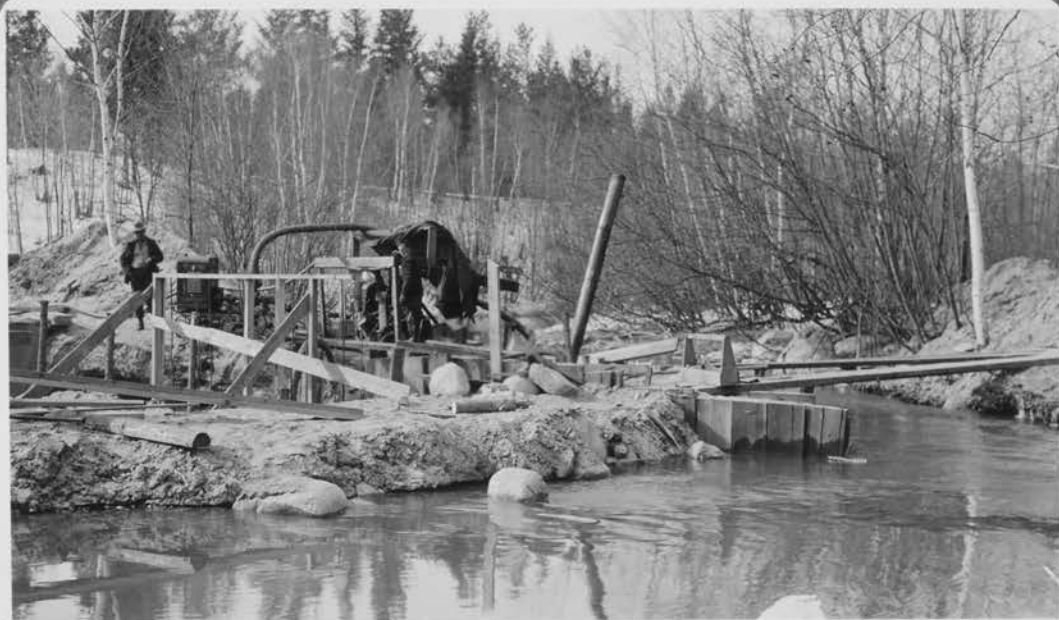
Temporary Earth Dam and Water by-pass
