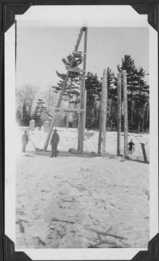
DRIVING PILING. BREAK WATER — KABETOGAMA RANGER STAT.
