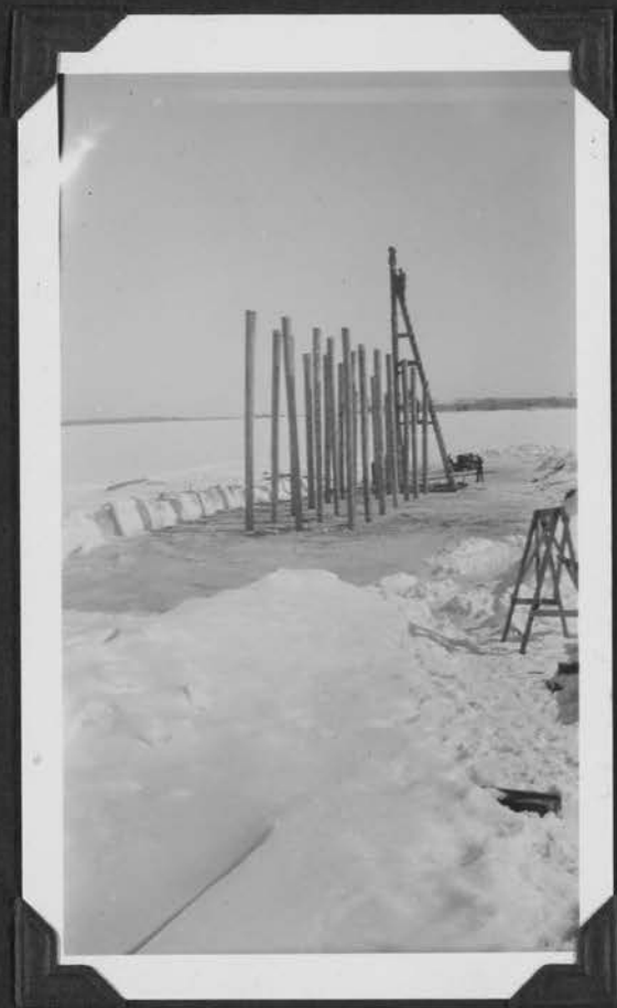
DRIVING PILING. BREAK WATER — KABETOGAMA RANGER STAT.
