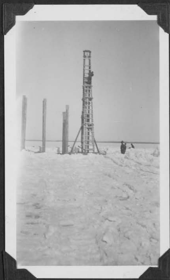
DRIVING PILING. BREAK WATER — KABETOGAMA RANGER STAT.
