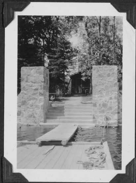
KABETO GAMA R. STATION FROM LAKE OLD BLDG IN BACKGROUND.
