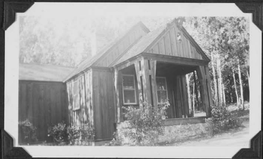
ASH RIVER TOWER CABIN
