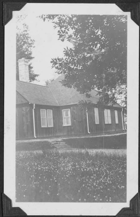
RANGER STATION SIDE & REAR
