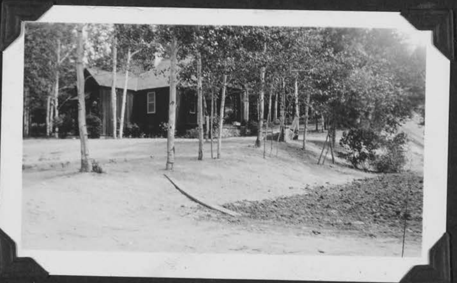
ASH RIVER TOWER CABIN
