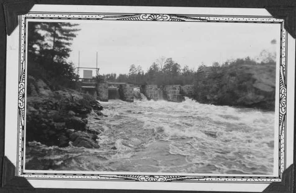
KETTLE FALLS DAM BELOW
