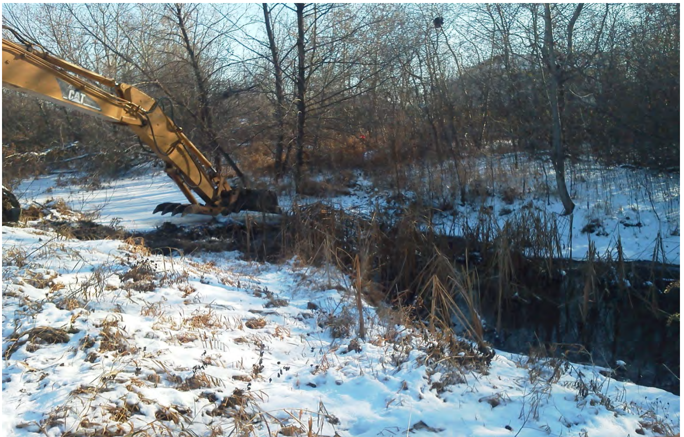
Beaver dam removal from ARJD #1 in Blaine winter 2011
