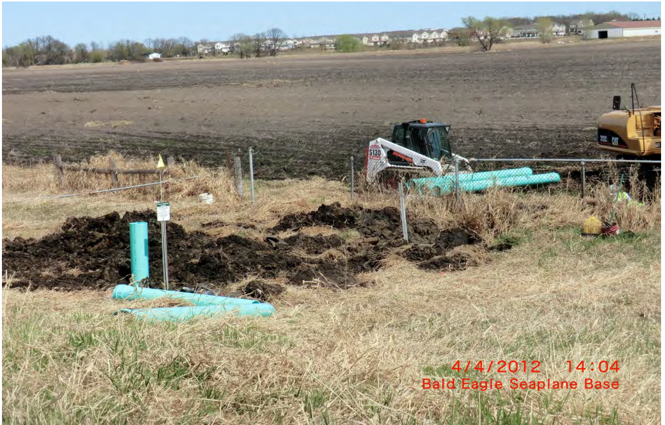
Tile Repair on ACD #55, Branch #8 (April 2012)
