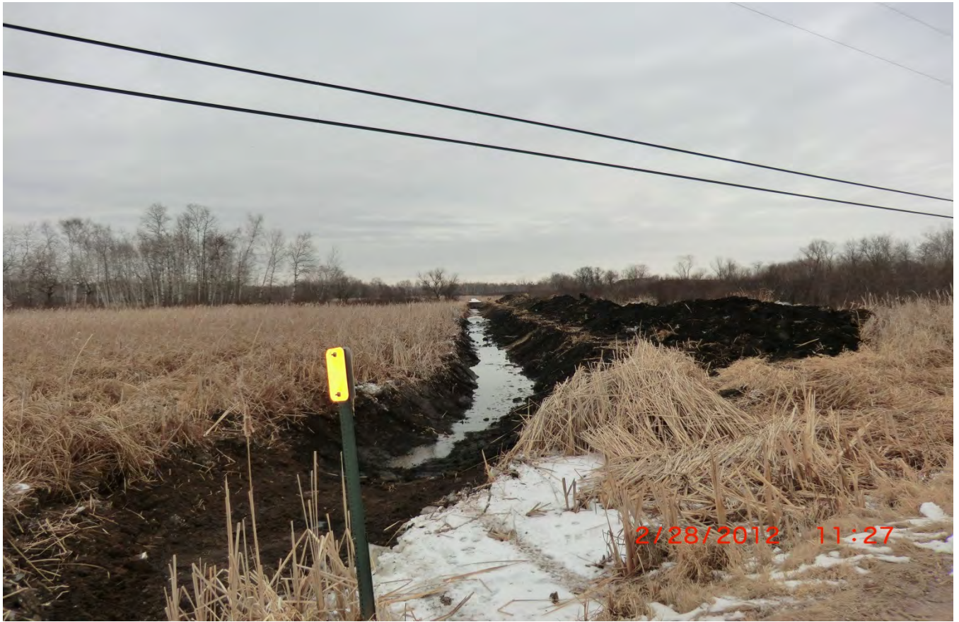
ACD #10-22-32 maintenance north of Pine Street February 2012
