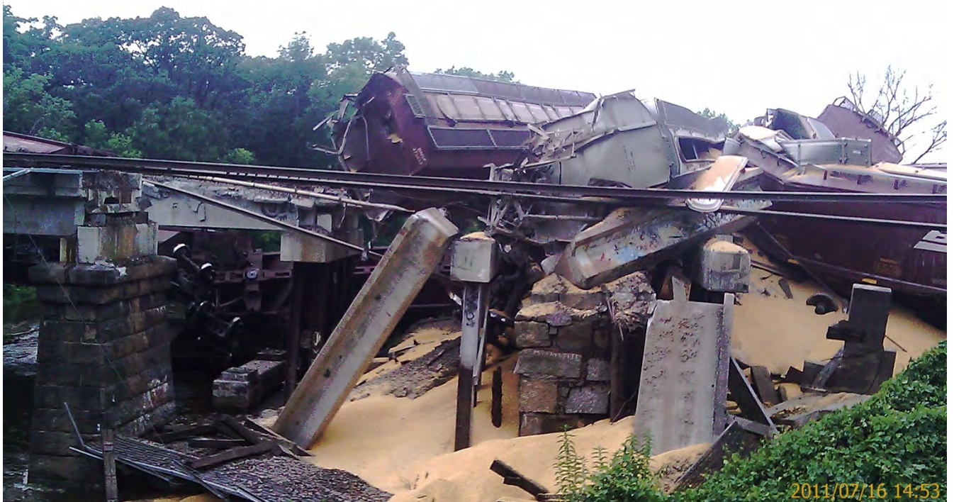
Train Derailment at Rice Creek crossing in Fridley (July 2011)
