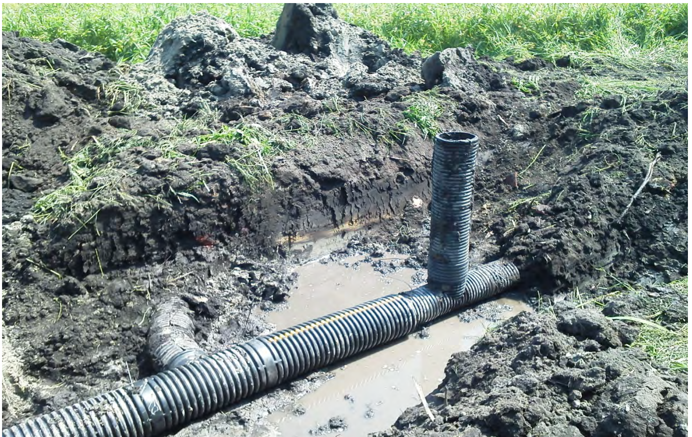
Tile Repair on ACD #55 main branch (July 2012)
