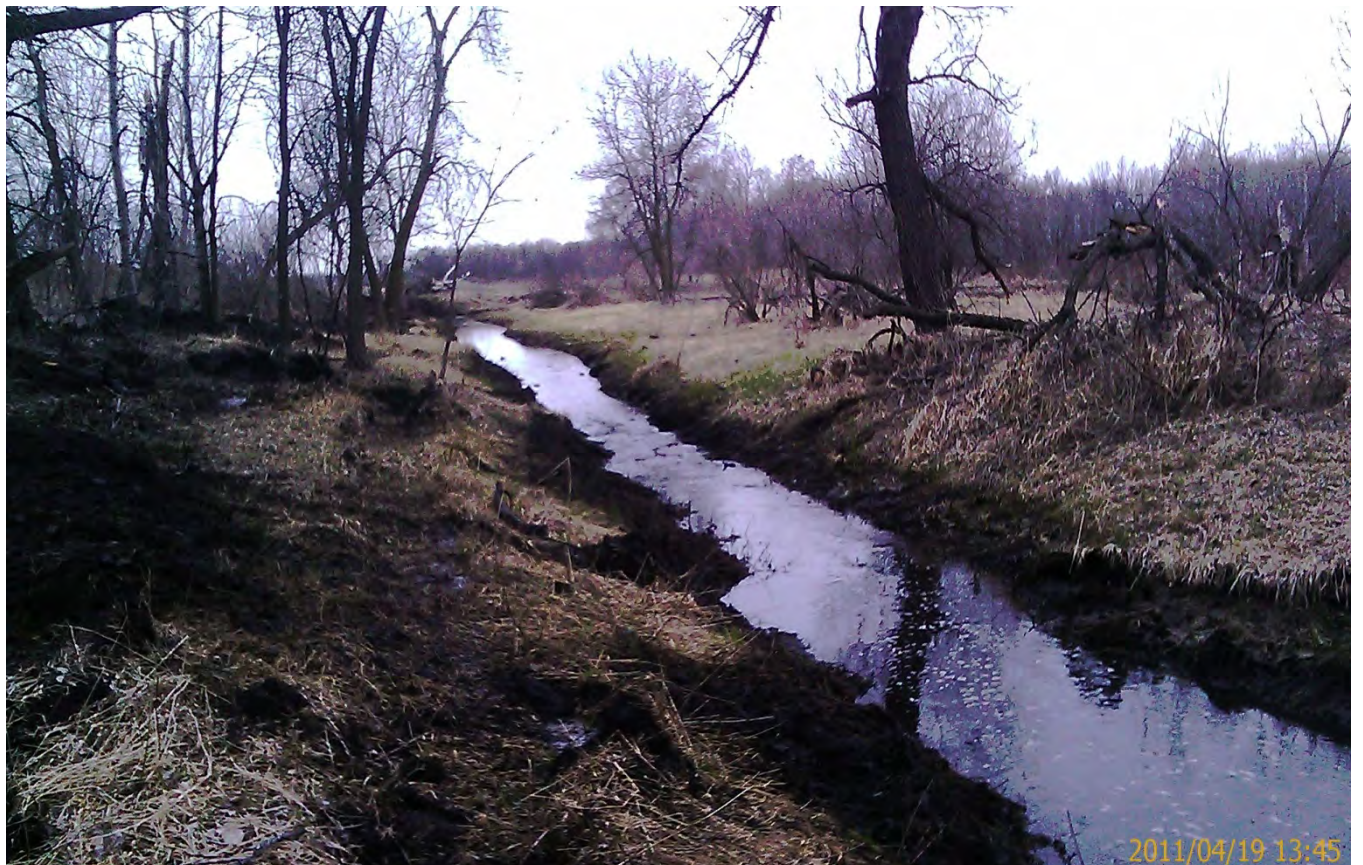
ACD 53-62 Branch #1 maintenance between Main St. and 121 st Ave 2011
