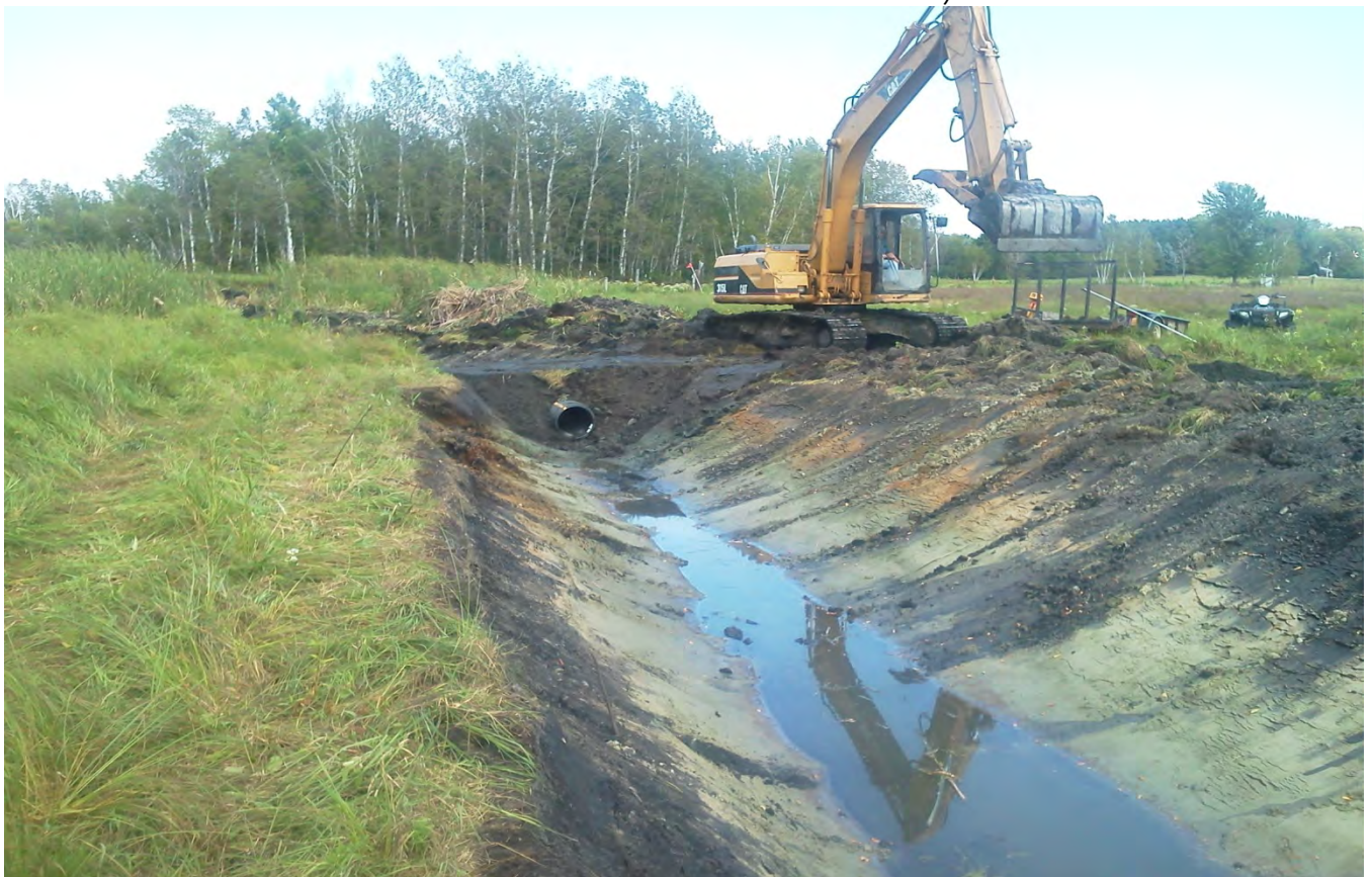
ACD #10-22-32 maintenance north of Pine Street September 2012
