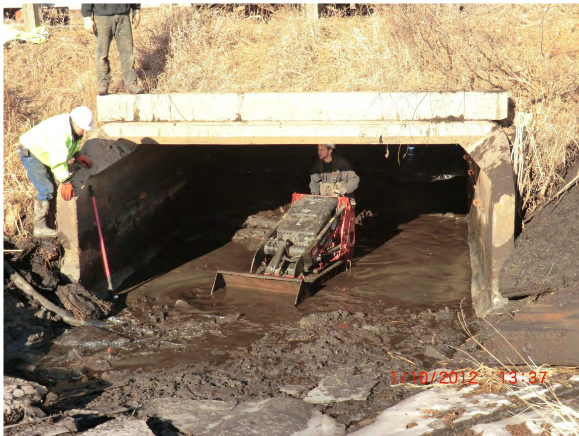
WJD #2 Maintenance at 165 th Street culvert in Hugo (January 2012)
