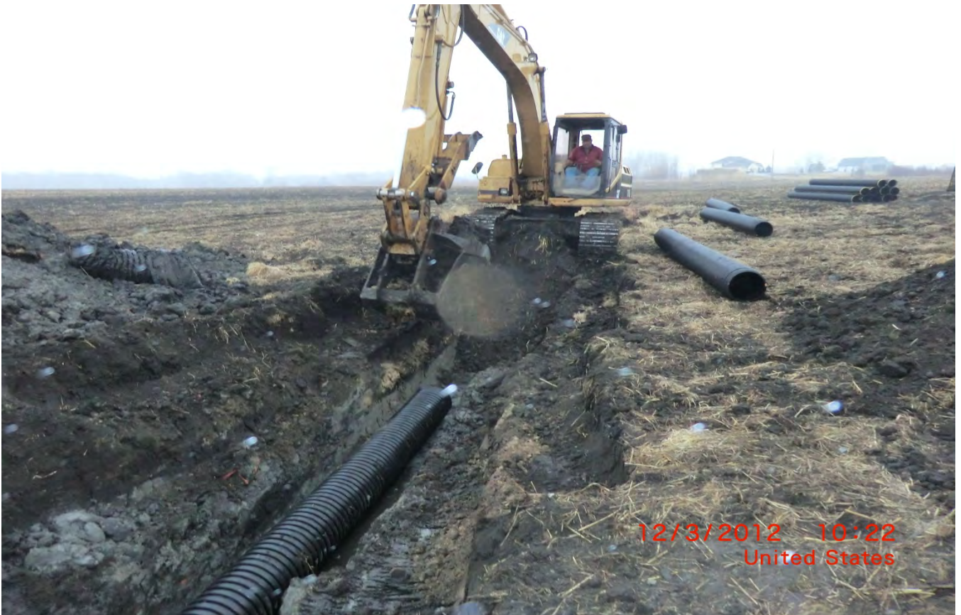
Tile Repair on AWJD #4, Branch #3 in Forest Lake (December 2012)
