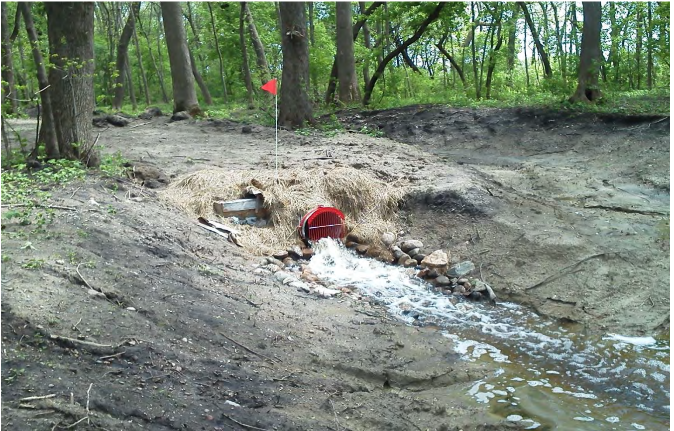
New tile outlet and headwall on AWJD #4, Branch #4 (March 2012)
