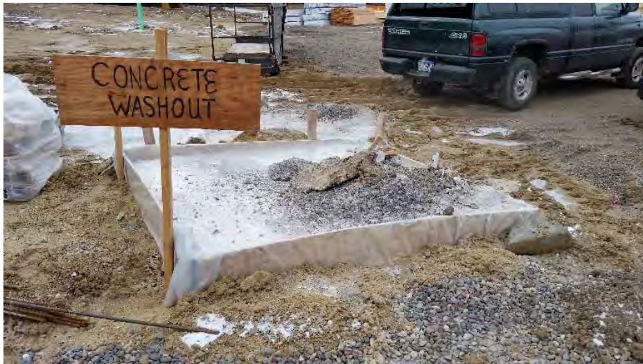
Photos: Underground filtration system piping (above) and concrete washout containment (below).
