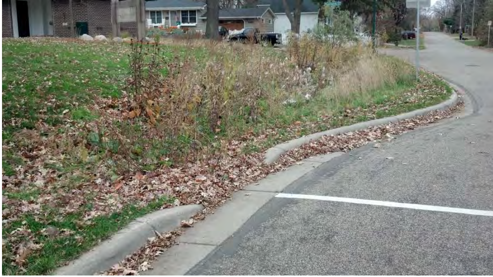
Photo: Leaf litter starting to accumulate at a curb cut inlet to a rain garden
