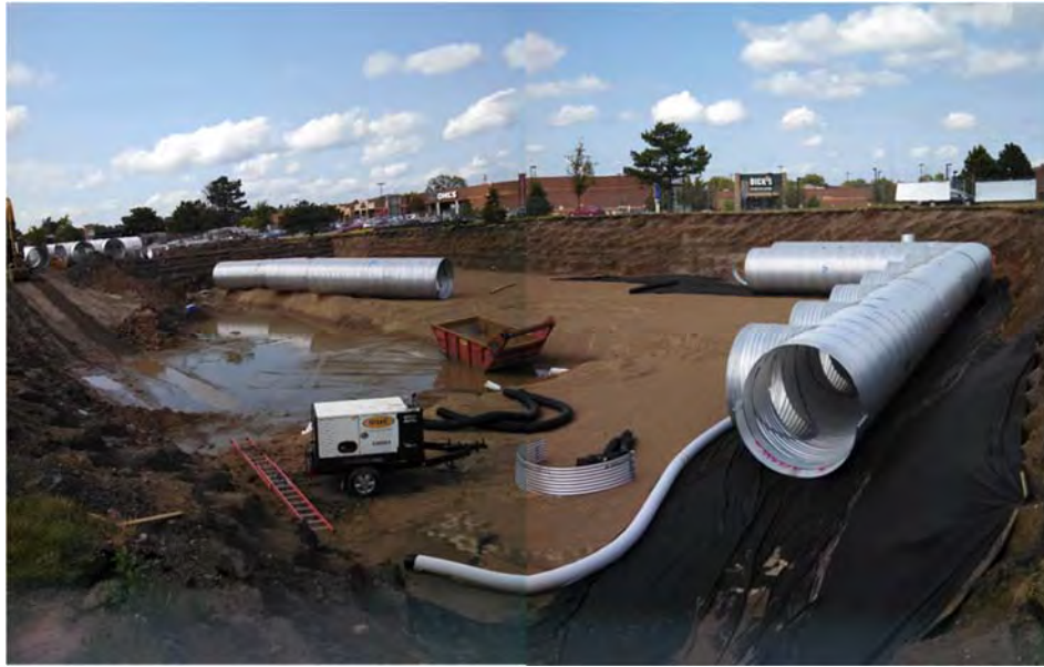
Photos: Underground filtration system piping (above) and concrete washout containment (below).
