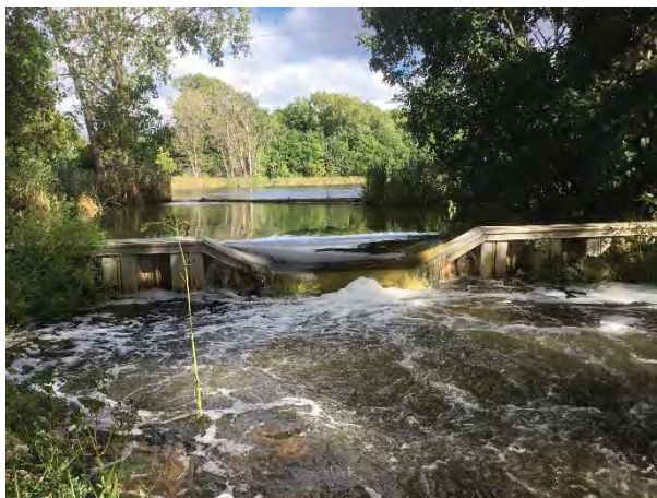
Photo at above: E2 Wetland Weir (09/2018)
