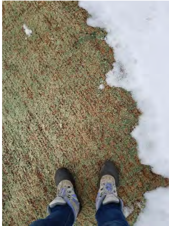
Above photo: Erosion control blanket with hydroseeding
