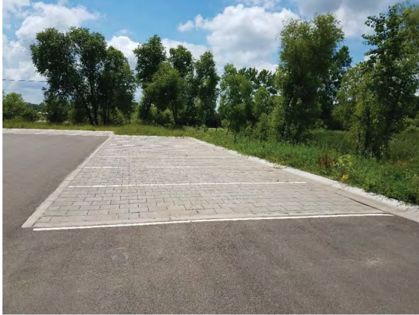
Above photo: Constructed permeable pavers in parking lot
