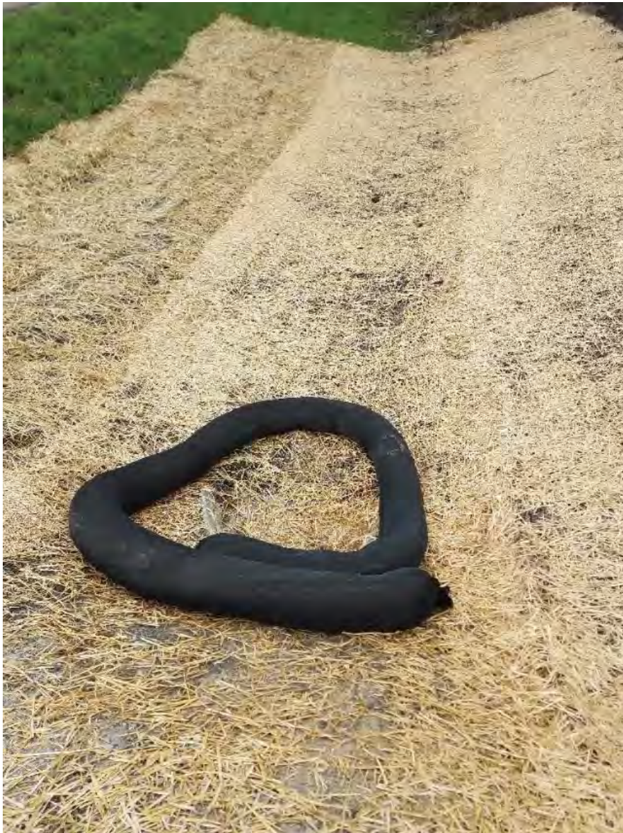
Above photo: Erosion and sediment control in a ditch bottom/driveway culvert
