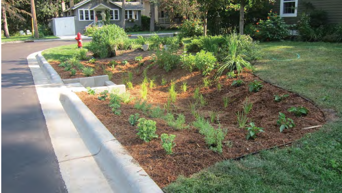
Two curb cut raingardens in White Bear Lake; part of the City's street reconstruction projects
