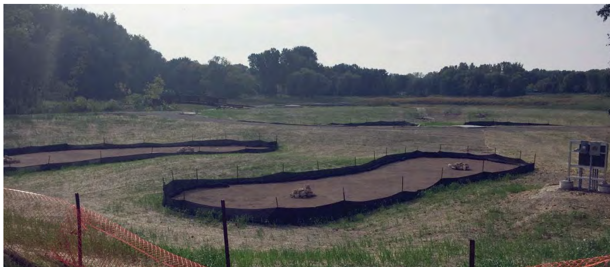
Iron-Enhanced Sand Filters under construction at Hansen Park
