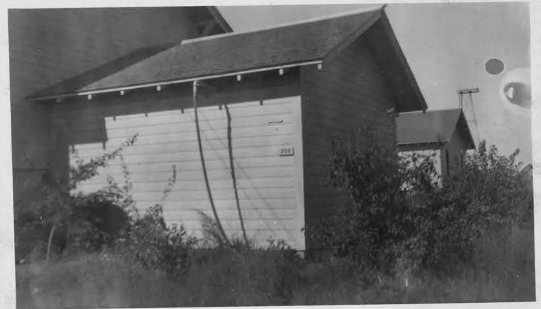
No. 250 Subject WELL HOUSE 5f36 Negative Print Slide Cut Taken by Place PARK RAPIDS Date AUG 1940
