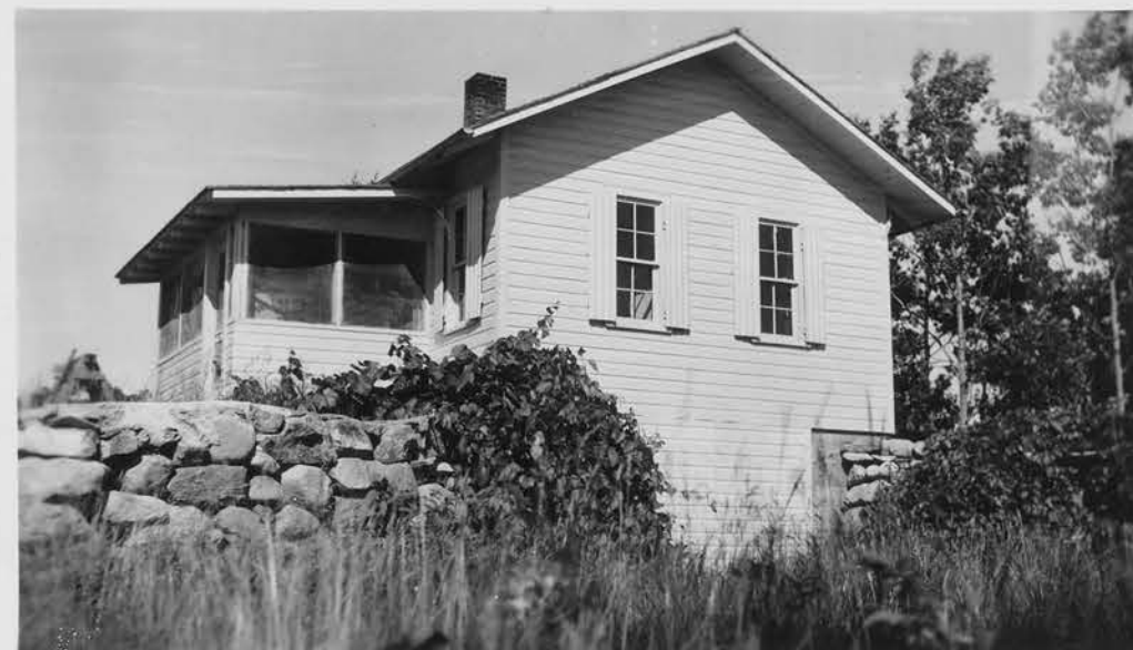
No. 57 Subject OLD PATROL CABIN FAS No 41 5F40 Negative ..... Print Taken by ..... ..... Slide Place MANTRAP VALLEY ..... Cut Date AUG 1940
