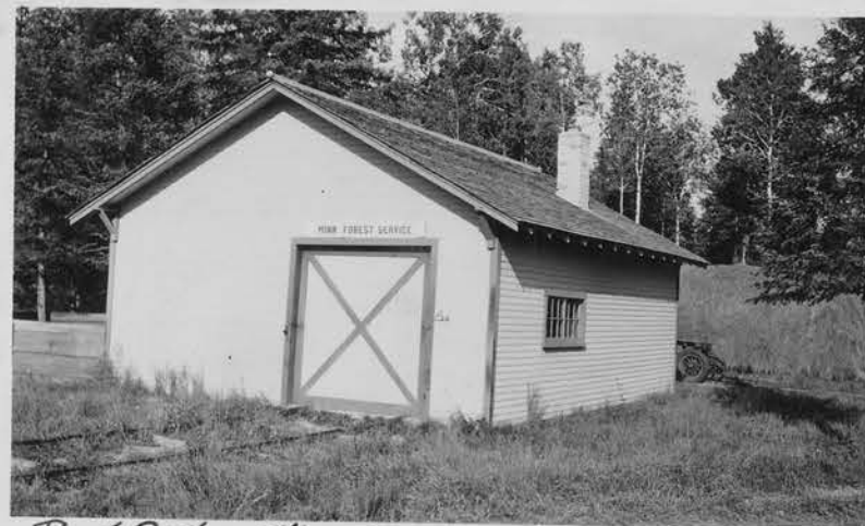
Rock Cut - Warehouse
