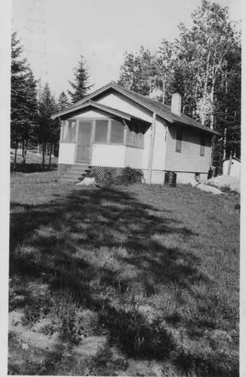
Rock Cut Ranger Station 9-4-40
