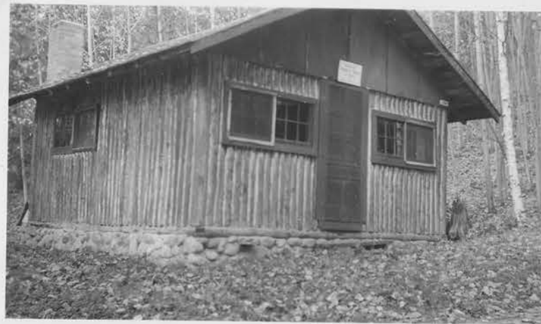
No. 220 Subject BUNK HOUSE
