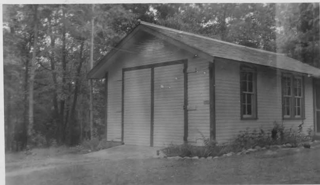
No. 256 Subject WARE HOUSE 5f182 Negative FCS NO 47 Print Slide Taken by Cut Place WOLF LAKE Date AUG 1940
