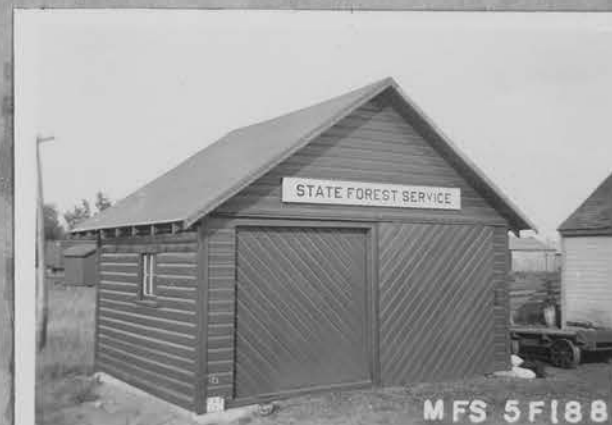
No. 241 Subject SPEEDER SHED 5f188 Negative FAS 231 Print Taken by Slide Place BEMIDJI Cut Date
