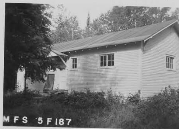
No. 609 Subject W.P.A. BUNK HOUSE 5f187 Negative FAS-118 Print Taken by Slide Place SEC11-148-33 Cut Date
