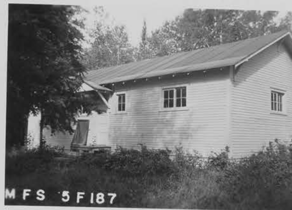
No. 609 Subject W.P.A. BUNK HOUSE 5f187 Negative FAS-118 Print Taken by Slide Place SEC11-148-33 Cut Date
