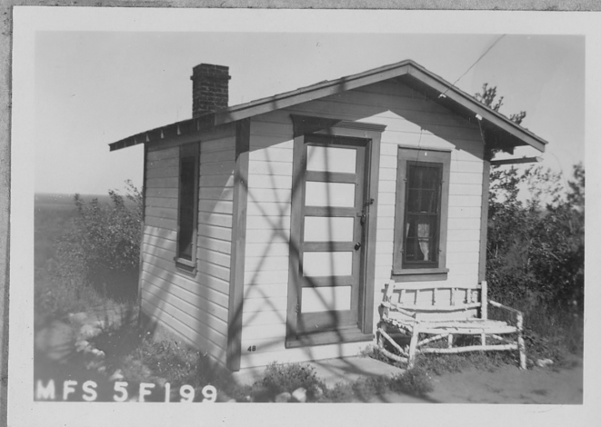
No. 48 Subject CABIN 5f199 Negative ..... Print Taken by..... ..... Slide Place LARAMOUNT-TOWER ..... Cut Date.....
