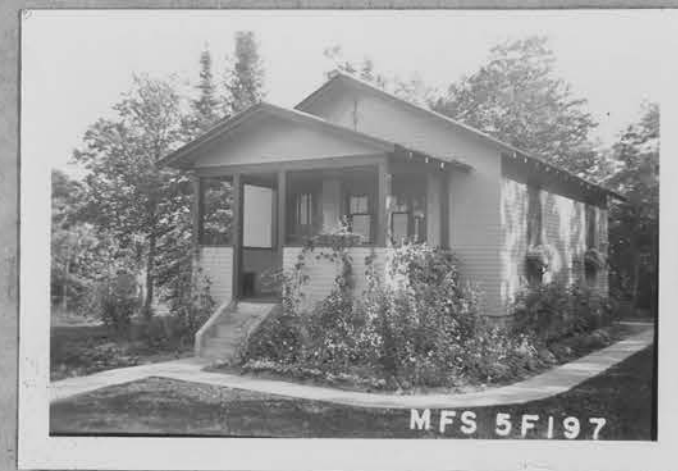
No. 49 Subject CABIN 5f197 Negative FAS # 28 ..... Print Taken by..... ..... Slide Place BUENA VISTA ..... Cut Date.....
