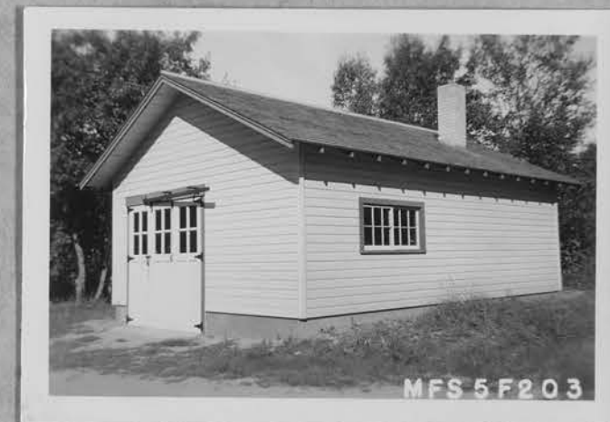
No. 239 Subject WAREHOUSE 5f203 Negative FAS 26 ..... Print Taken by ..... Slide Place LARS MOUNT ..... Cut Date
