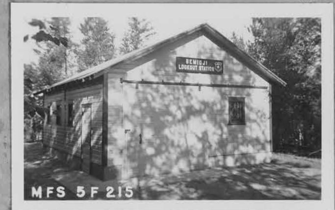
No. 243 Subject WAREHOUSE 5+215 Negative Print Slide Cut Taken by Place BEMIDJI Date
